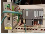
Local PROFINET network (left, short deterministic cycle time) and connection to remote sites and the cloud (orange frame, Internet communication).
