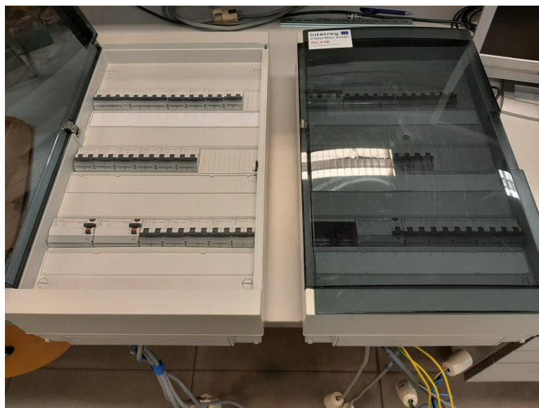
Fig. 2. Connection box house
