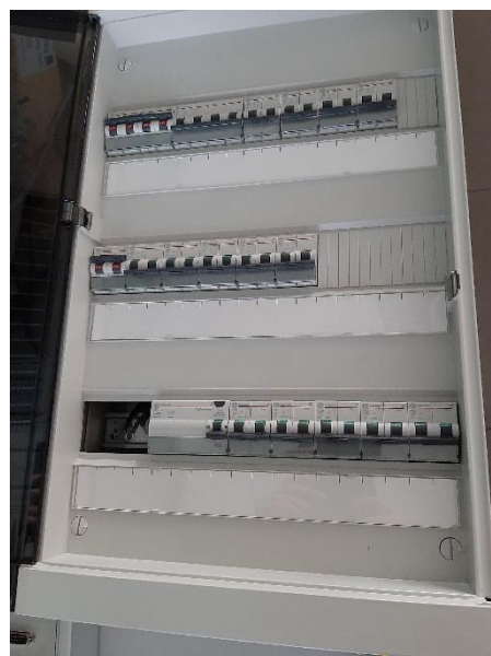
Fig. 2. Connection box house
